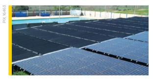
Integrated solar hot water and photovoltaic panels offset energy consumption for heating and pumping systems at the Camp Pendleton Area 62 training pool.
