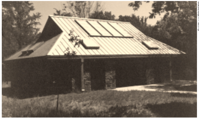
The solar hot water system on this small comfort station at Chickasaw National Recreation Area supplies all the hot water for the building. There is no backup system.
