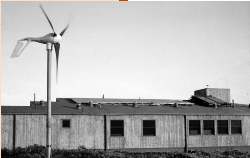
A hybrid wind/PV energy system powers the ranger station on San Miguel Island.
