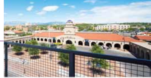
The apartments are across from the Alvarado Transportation Center, a regional transit hub.
