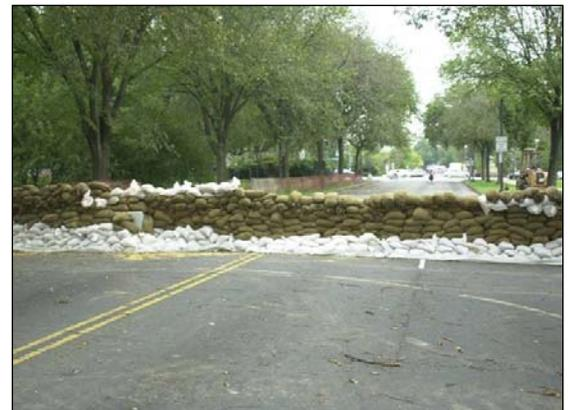
N.W., between the levee and the Washington Monument. These procedures involve bringing in “Jersey barriers” and sand bags, as well as removing soil from the Washington Monument grounds to build a temporary earthen levee. They are labor intensive and not completely reliable. Post-Katrina federal standards require a more reliable levee system be in place.
