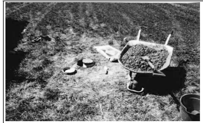
Figure 8.26. Mixing concrete for use in completing the monument.
