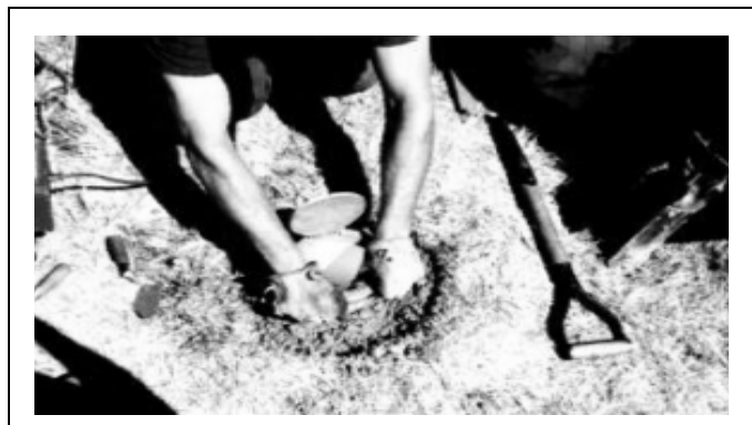
Figure 8.27. Shaking the PVC pipe to settle concrete and fill any voids.
