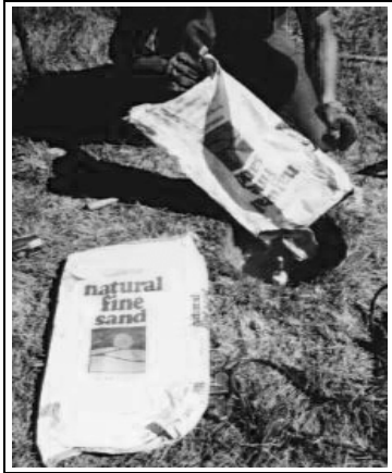
Figure 8.24. Backfilling the bottom two feet of the hole with washed sand
