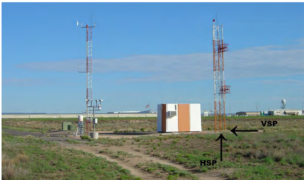
Figure C-6. Typical glideslope installation.
