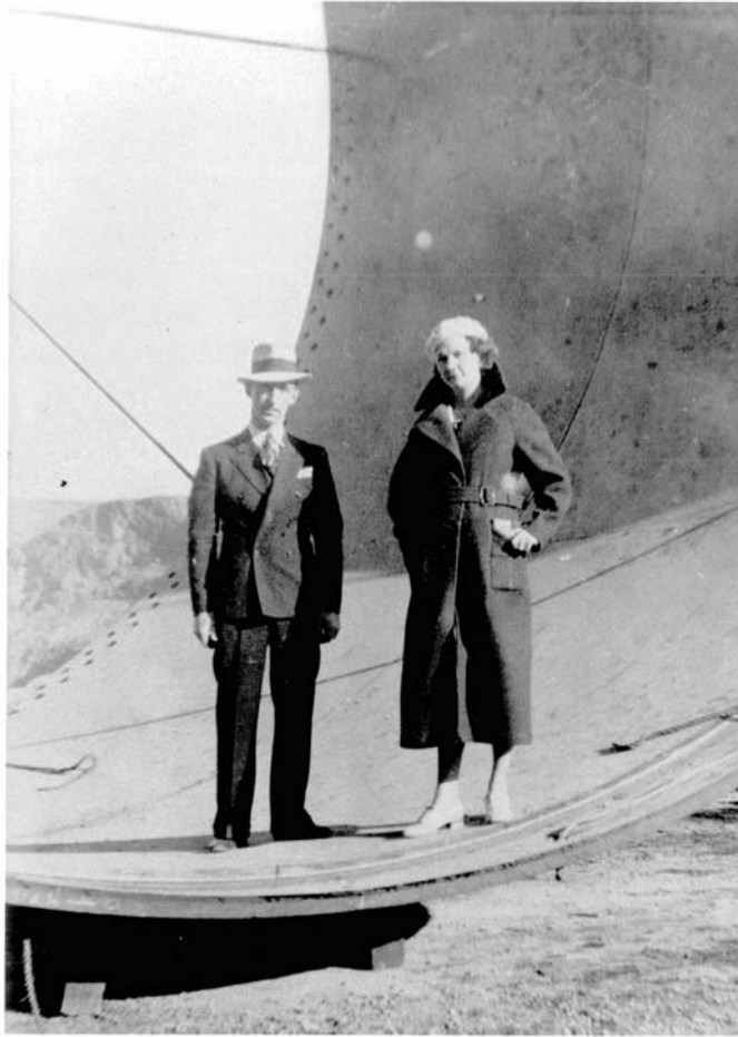
Illustration 11: Mr. and Mrs. Charles Kelly Sweet standing in a 30' diameter penstock section ready to be moved via cableway for use at Hoover Dam.
