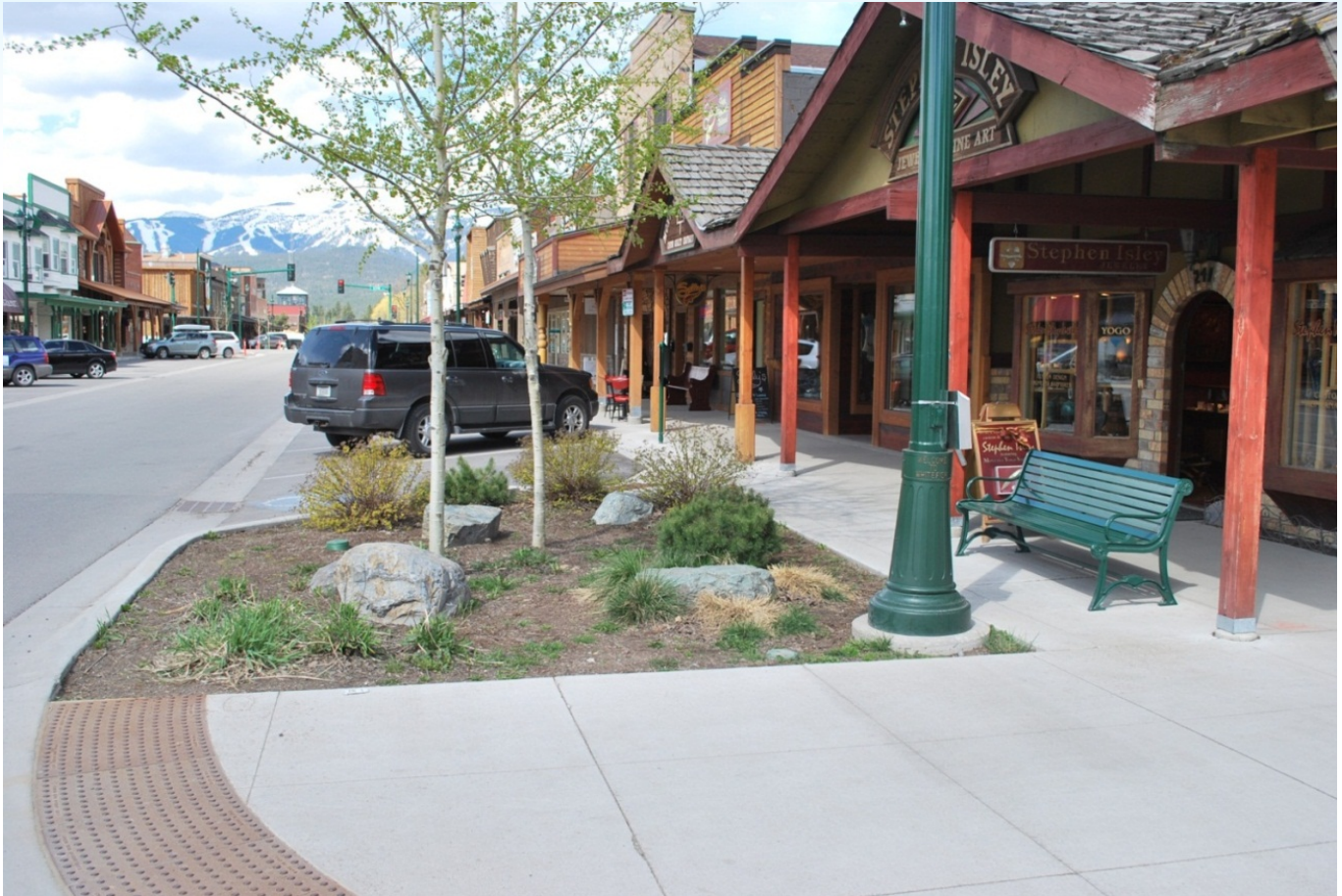
Figure 2: The U.S. Highway 93 2 nd Street Improvement Project brought many new pedestrian-friendly amenities to downtown Whitefish, Montana.
