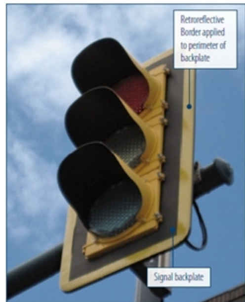
Figure 6: A yellow retroreflective border on a signal backplate.
