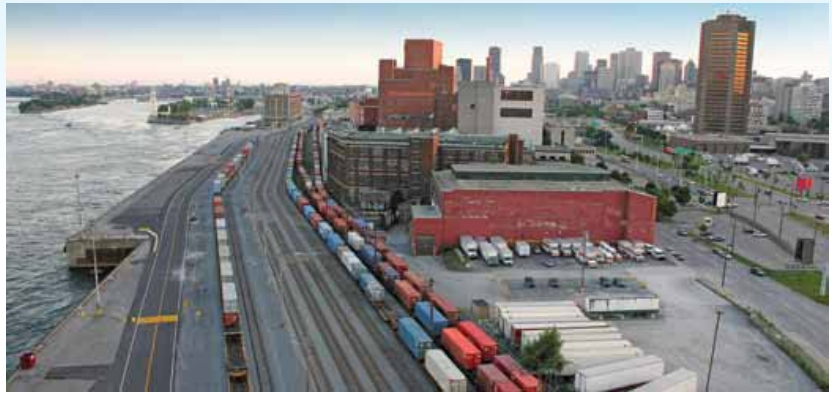
Figure 1: This freight rail facility in Montreal, Canada abuts commercial and residential areas.
