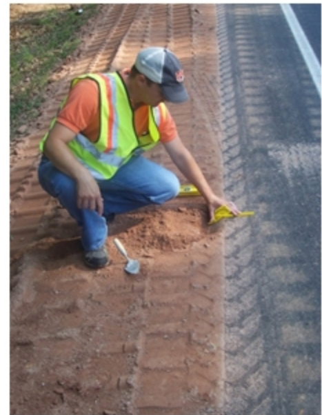
Figure 4: The angle of a Safety Edge SM can be measured before or after shoulder grading is complete.
