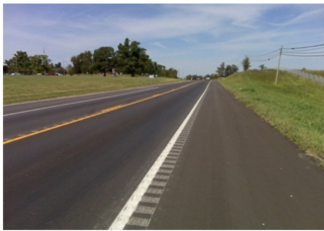
Figure 5: Rumble strips warn inattentive drivers if their vehicle leaves the travel lane.
