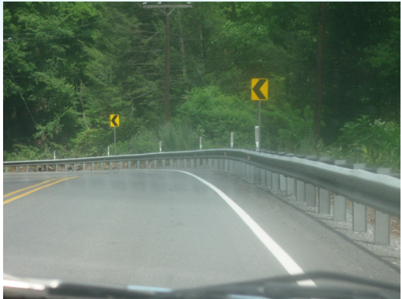
Figure 3: Chevrons, delineators, and pavement markings warn drivers of an impending curve on a rural roadway.
