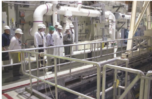
Spent Fuel Pool
