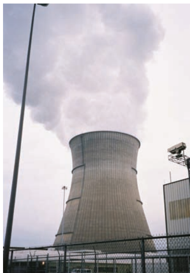
Natural Draft Cooling Tower
