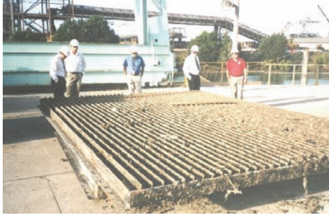
Intake Trash Bars
