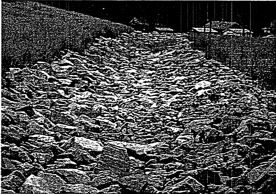
Figure F-2. Marginally-placed riprap
