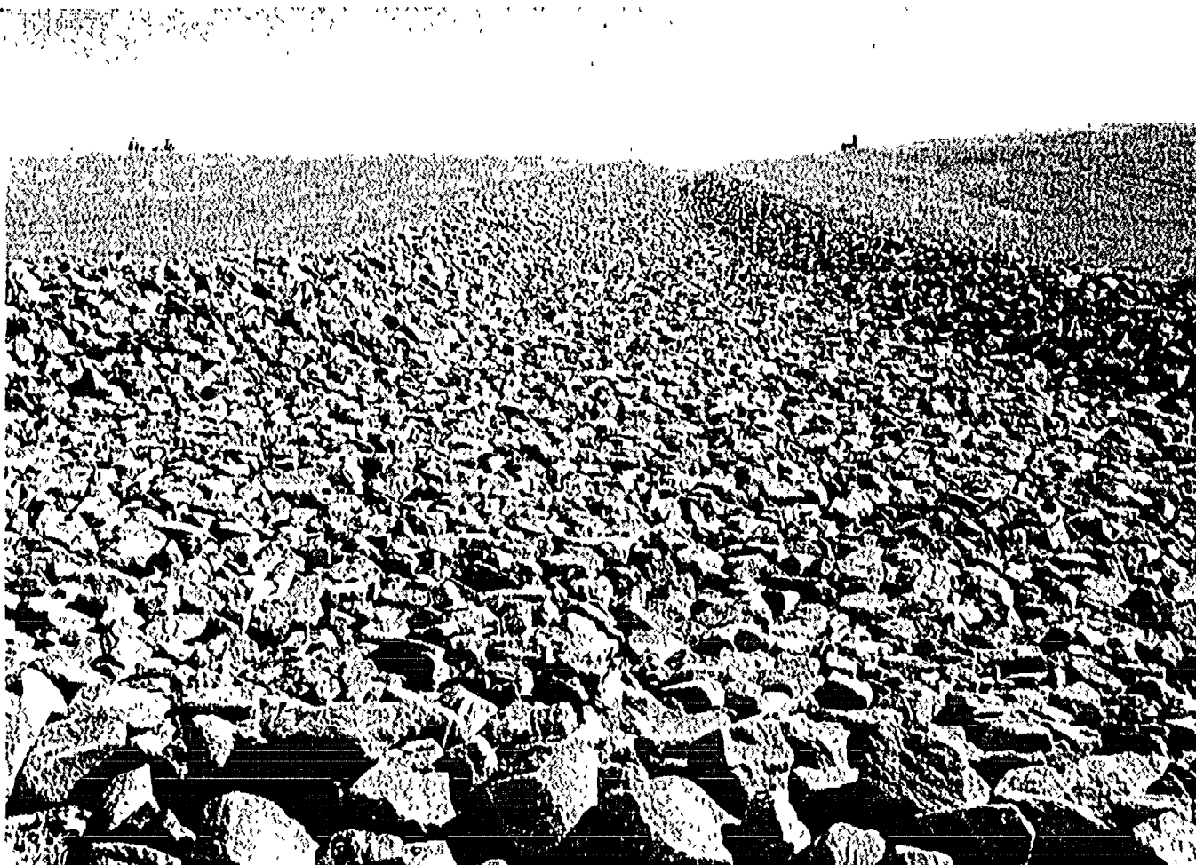
Figure F-5. Well-placed riprap in diversion channel.
