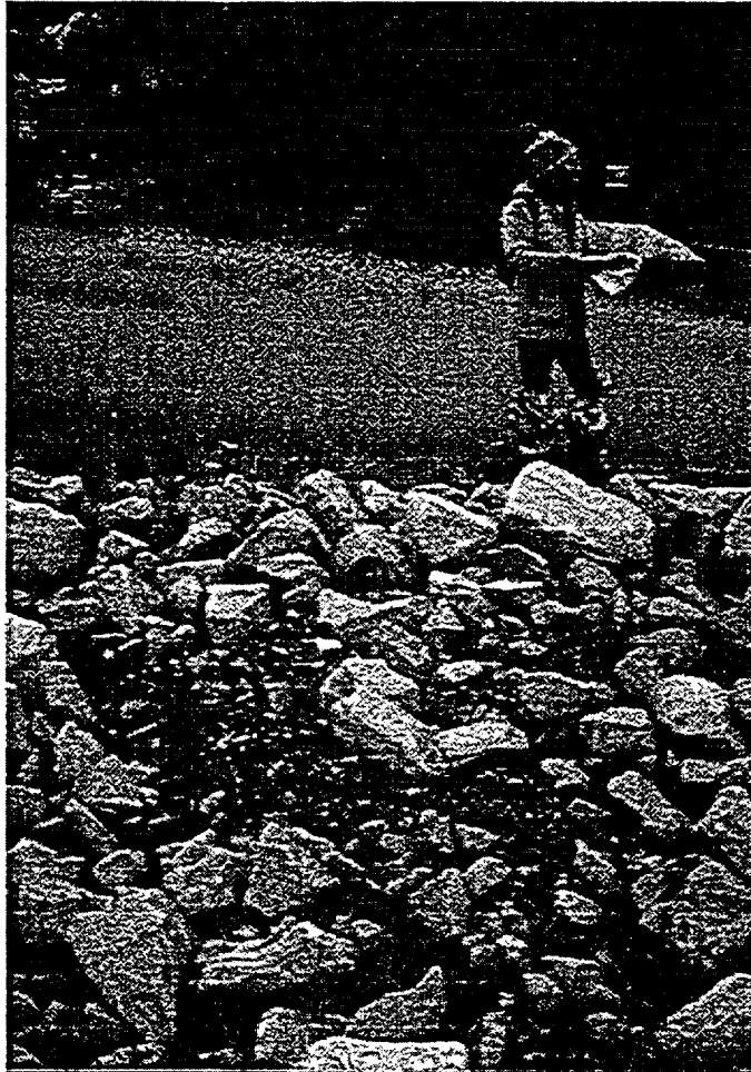
Figure F-1. Poorly-placed riprap.
