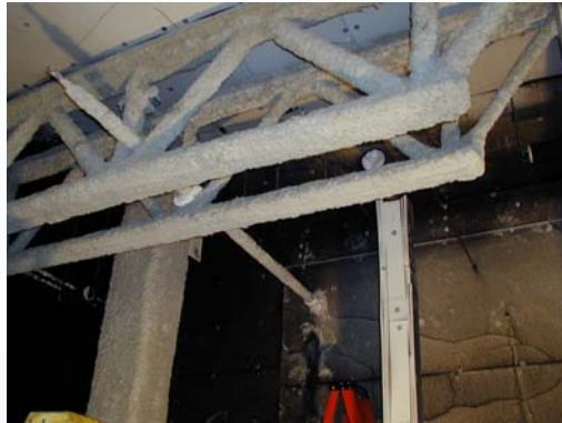
Prediction of steel temperatures through fireproofing
