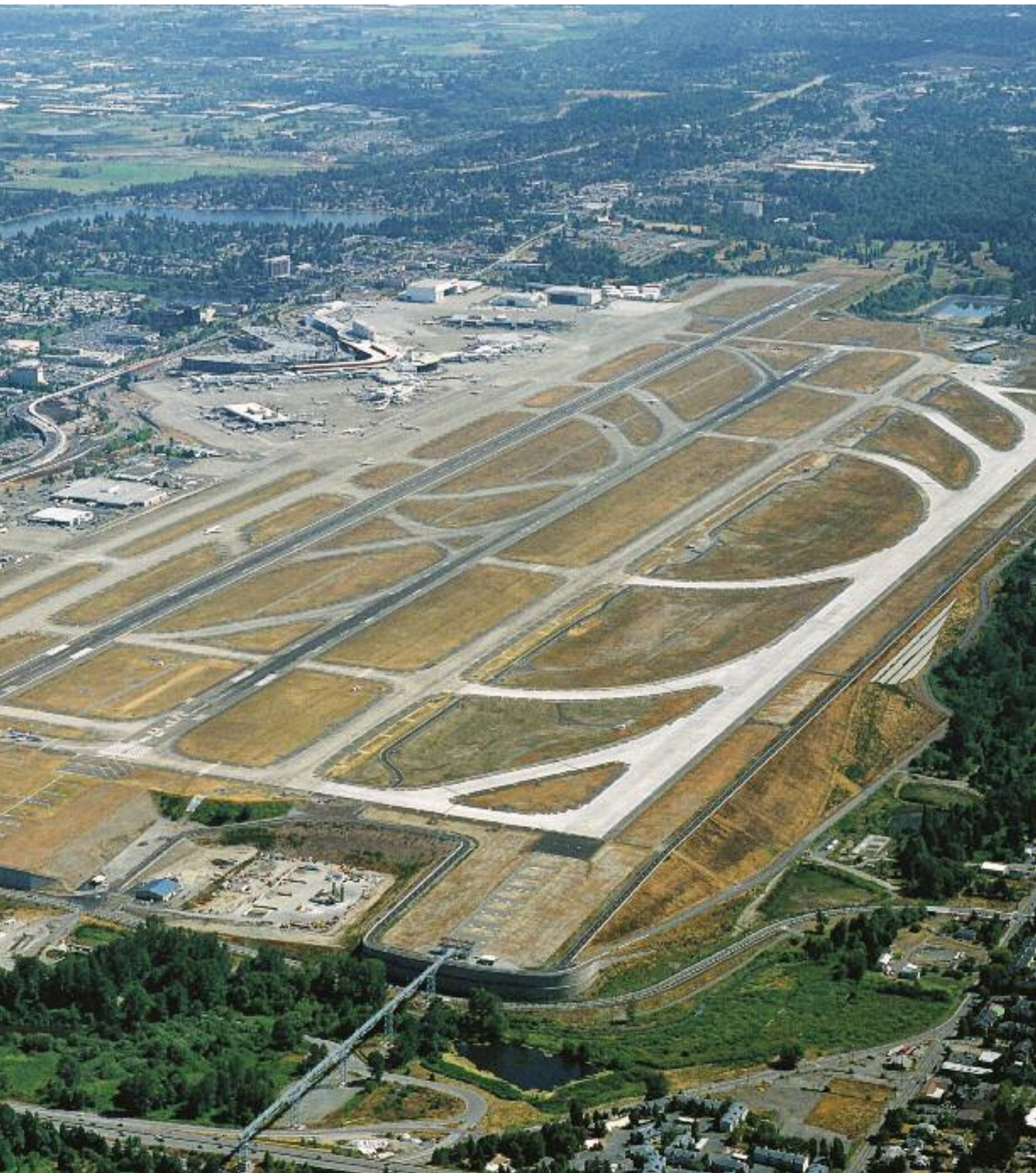
Photo: Construction of the Seatac 3rd Runway © 2008 Sky-Pix
