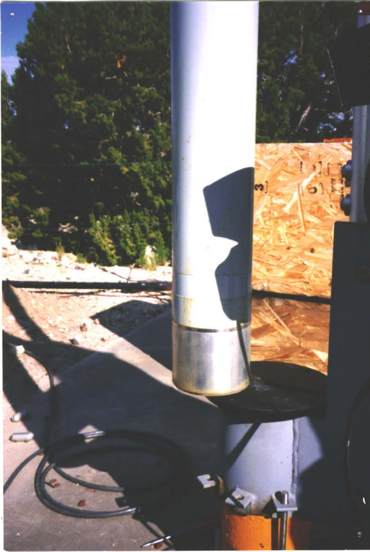
Bottom end of KS-54000 assembly with the "sand foot" installed".
