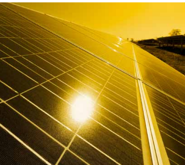
Abu Dhabi's US$600-million solar power plant, expected to be complete in 2012, will be one of the largest concentrated solar power plants in the world. © Fernando Alonso Herrero
