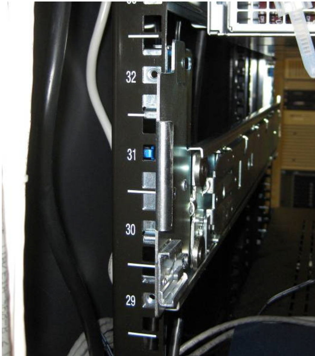
Figure A-6: R900 Rail Installed - Rear of Rack
