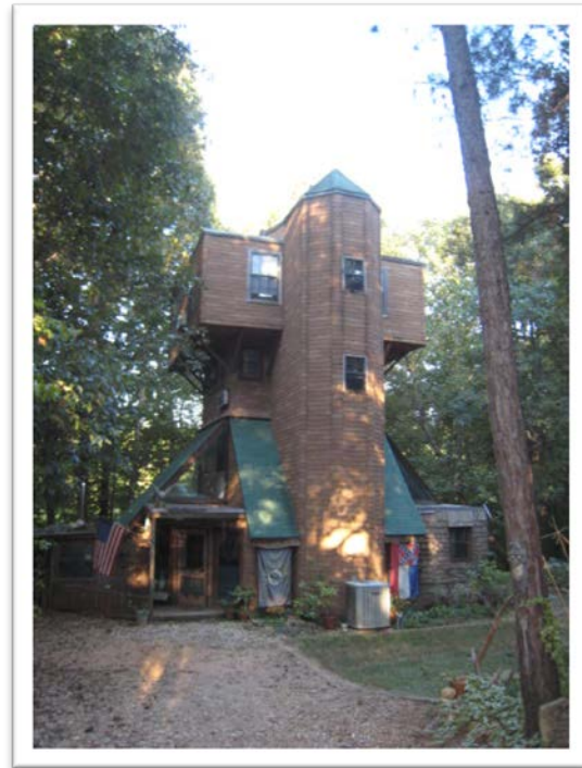
A residence impacted by the State Route 9 project (source: MDOT)
