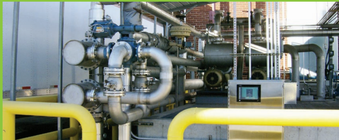
Based on recommendations from their Save Energy Now assessment, Shaw Industries plant #20 in Dalton, Georgia, installed a waste water heat exchanger on their Kuster dye line to capture excess heat and save a significant amount of money and energy.
