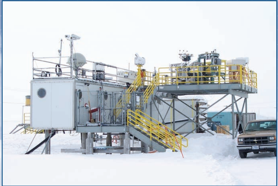
The ARM Climate Research Facility’s “Great White” instrument shelter was installed in Barrow in 1997. The Sky Deck, surrounded by yellow rails, was added to support additional instrumentation. ARM has a second research facility in Alaska located approximately 70 miles south of Barrow in the city of Atkasuk.
