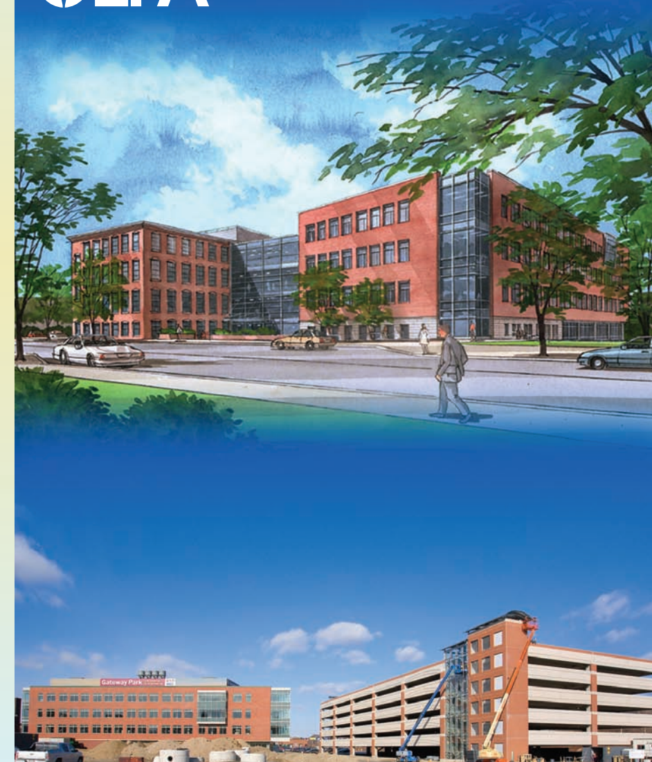
The Gateway Park redevelopment project in Worcester, Massachusetts, creating more than 1.5 million square feet of commercial space.
