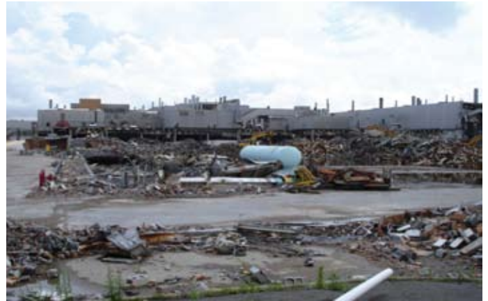
Demolition of the former GM Baltimore Plant
