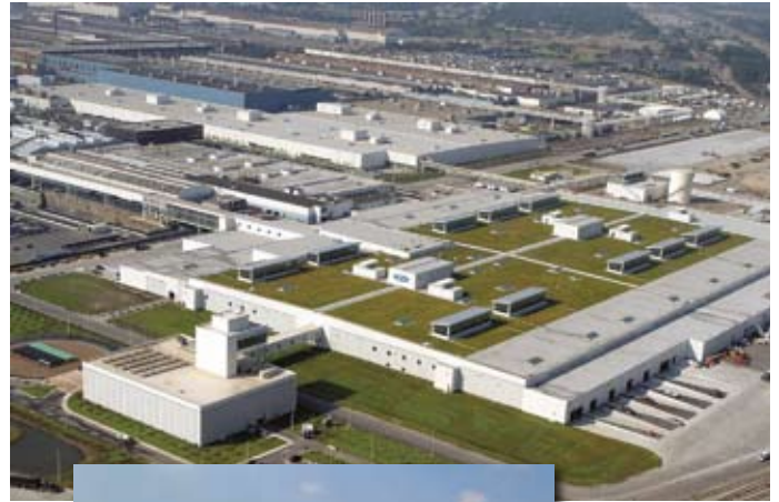
Aerial view of the Ford Rouge Plant's green roof
