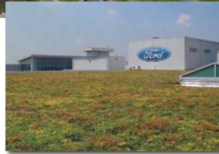
Ford's sustainable green roof is composed of nine varieties of sedum
