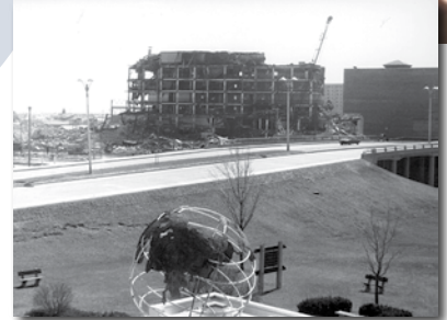
Demolition of the Former Chrysler Plant
