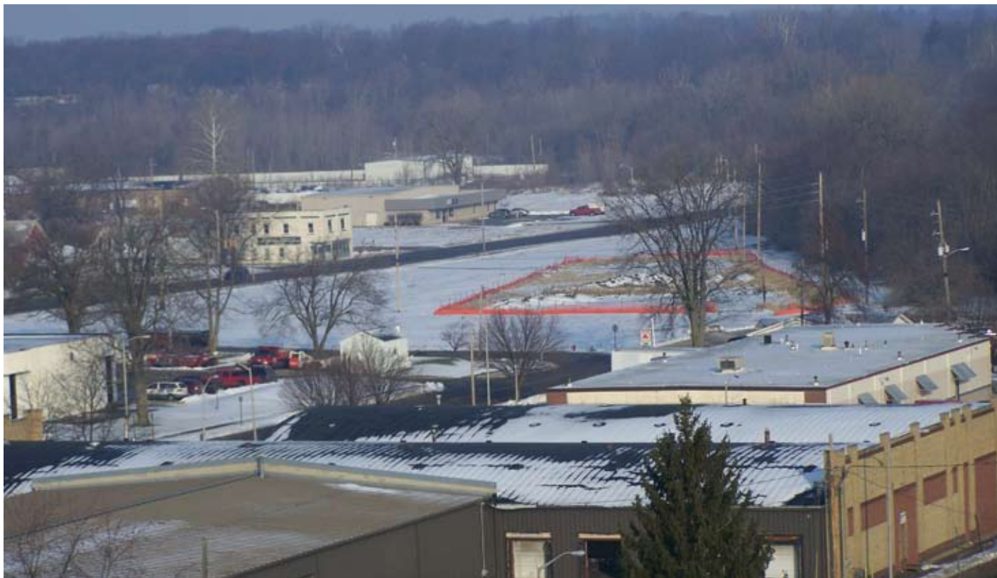
Prime Battery site after demolition activities
