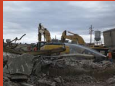
Demolition at Gates Rubber Plant, Denver, CO
