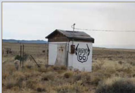
Abandoned outbuilding along Route 66
