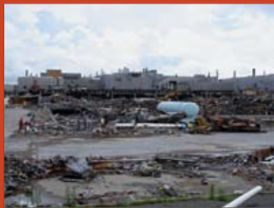
Former GM plant, Baltimore, MD
