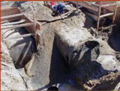
Underground Storage Tank removal
