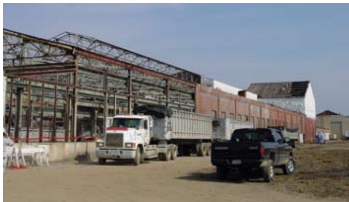
Construction activities at the former PPG Factory
