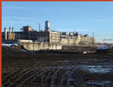
Denver, CO manufacturing plant
