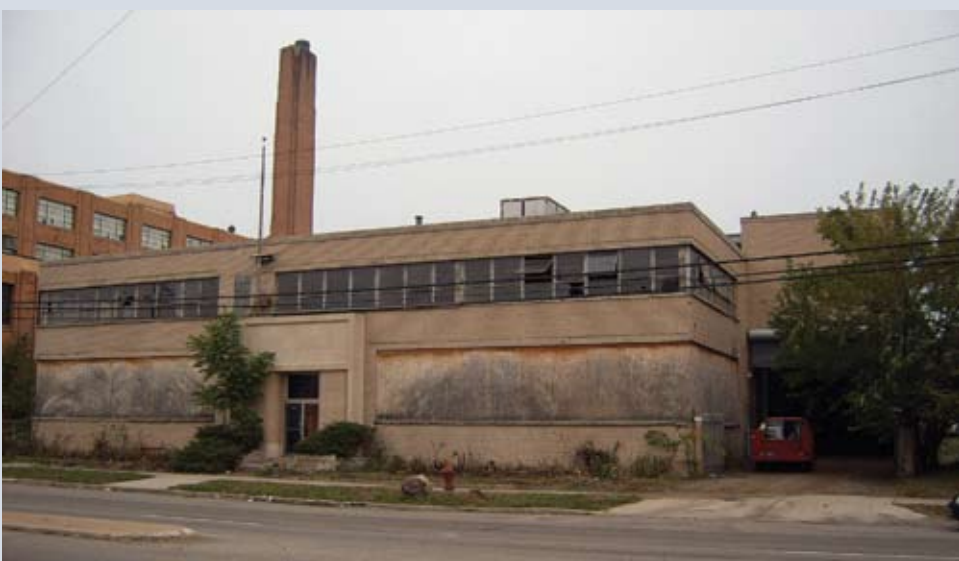
The Federal Engineering Building before cleanup and demolition activities
