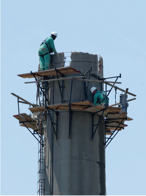
The smokestack that served ORNL's original steam plant was dismantled piece by piece earlier this year.
