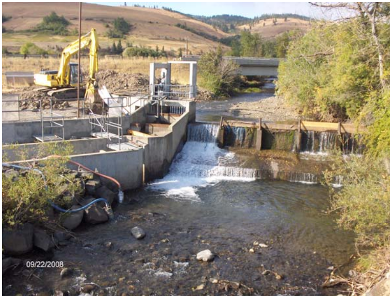
Figure 2. Bruton Dam at high and low creek flows. The fish ladder is to the left; Interstate-90 bridge is in the background.
