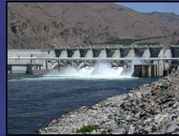
Rocky Reach Dam
