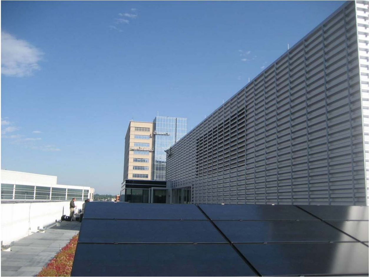
Figure 1. Roof sampling location.
