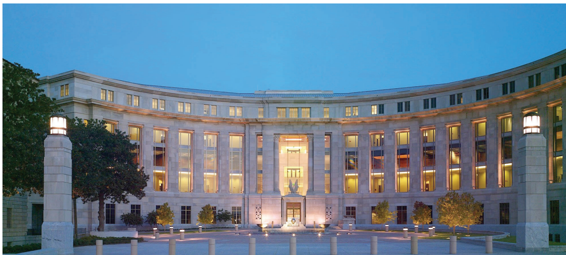
Frank M. Johnson Annex, Montgomery, AL
