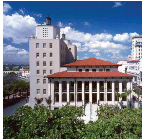
Jose V. Toledo Federal Building and Courthouse, Old San Juan, Puerto Rico
