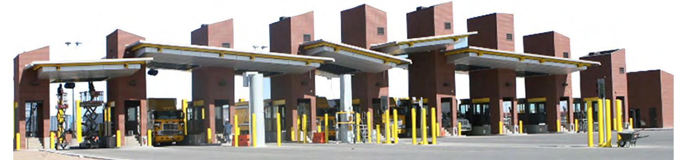
Ysleta Port of Entry El Paso, TX
