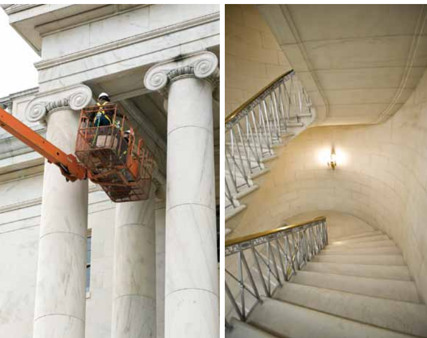
LEFT: The House Office Buildings jurisdiction provides the daily domestic care, structural and equipment maintenance for the U.S. House of Representatives' office buildings. In this photo, workers conduct a stone survey and repair at the Longworth House Office Building. MIDDLE: The AOC cleared an Office of Compliance citation by constructing enclosures for the four main egress stairs in the historic Longworth House Office Building. RIGHT: Due to an innovative redesign and team partnering on the Rayburn House Office Building roof replacement project, the AOC was able to meet the original design intent with a substantial cost savings for the government.
