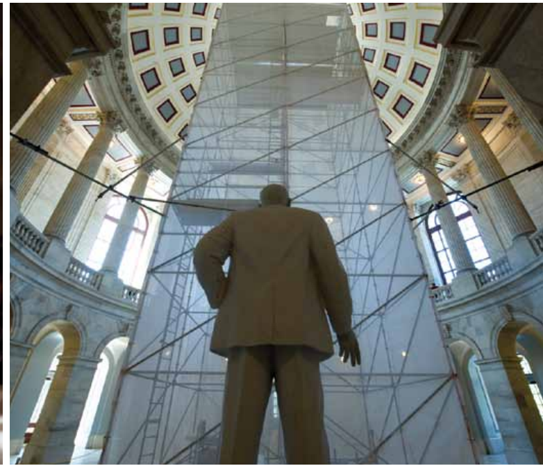
LEFT: In Senate Appropriations Room S-127 of the U.S. Capitol, conservators removed yellowed varnish and overpaint from the lower walls the room, restoring the vivid colors and definition of artist Constantino Brumidi’s cherubs and pilasters. RIGHT: A skylight replacement project in the Russell Senate Office Building began in the closing months of FY 2010 to eliminate leaks and improve energy efficiency. Construction requires scaffolding in order to replace the lay lights and repair the areas around the skylights.
