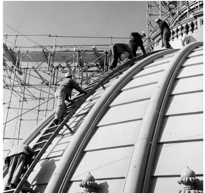
ABOVE: The last significant exterior renovation of the U.S. Capitol Dome, shown above, was performed in 1959 and 1960 when the ironwork was stripped of its paint so it could be primed with a rust inhibitor. LEFT: The octagonal fountain between the U.S. Capitol’s grand stairs was added to the Capitol terrace in 1889. Today, the AOC’s stewardship responsibility covers the maintenance and upkeep of this and other heritage assets.
