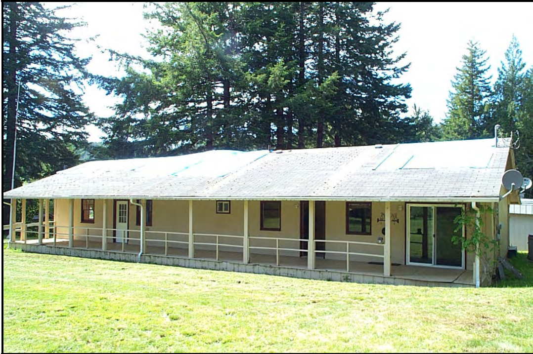
Bunk House building has three units.
