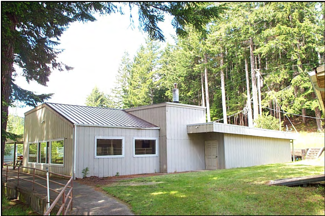
Looking north at the main lodge building.
