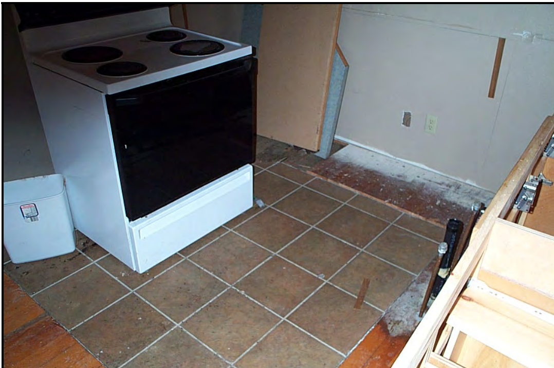
Kitchen area is partially remodeled.
