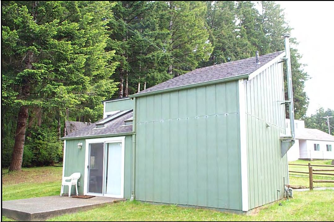
Looking east at cabin building, this one has been remodeled.
