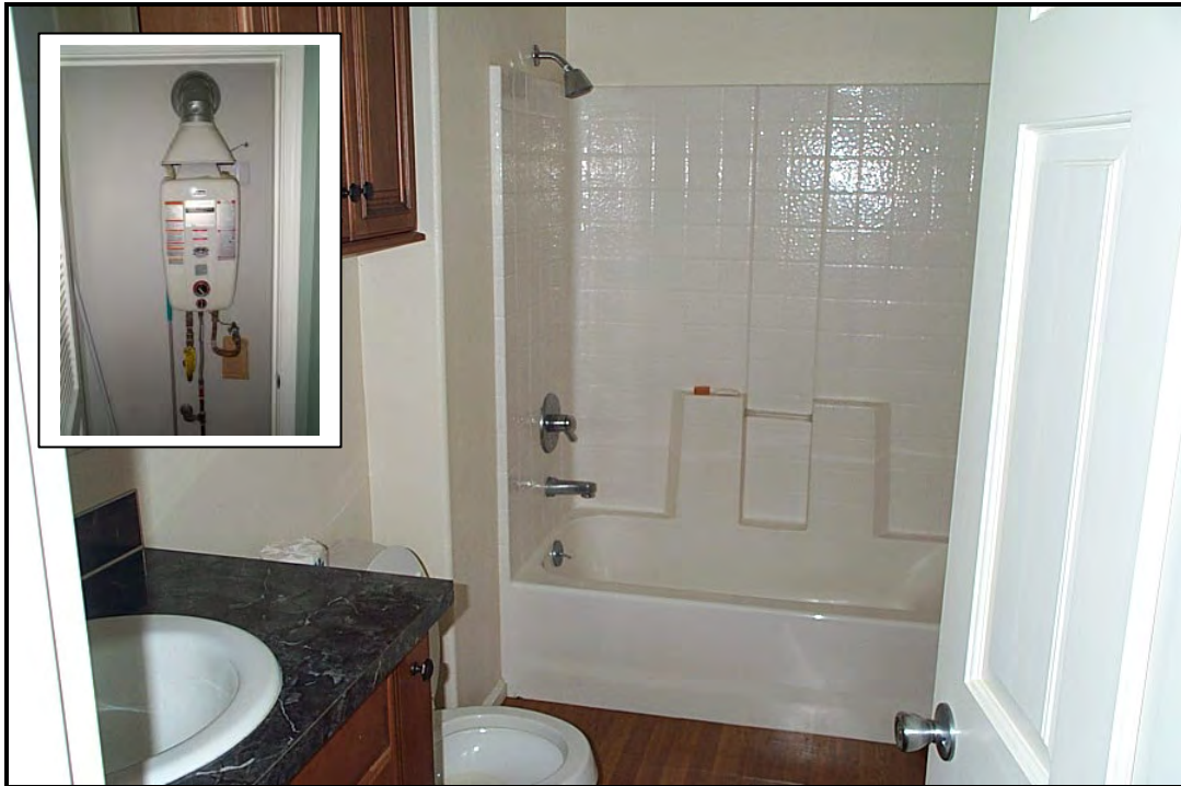
Remodeled bathroom with insert of the hot water heater used in all remodels.
