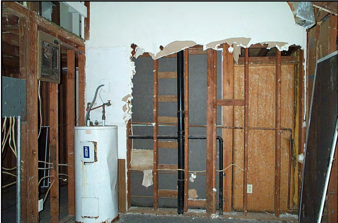
Interior view with old hot water heater and stripped down walls.
