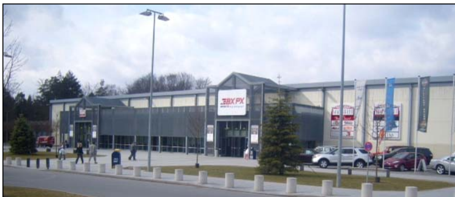
The new Main Exchange at Panzer Kaserne, Stuttgart.
