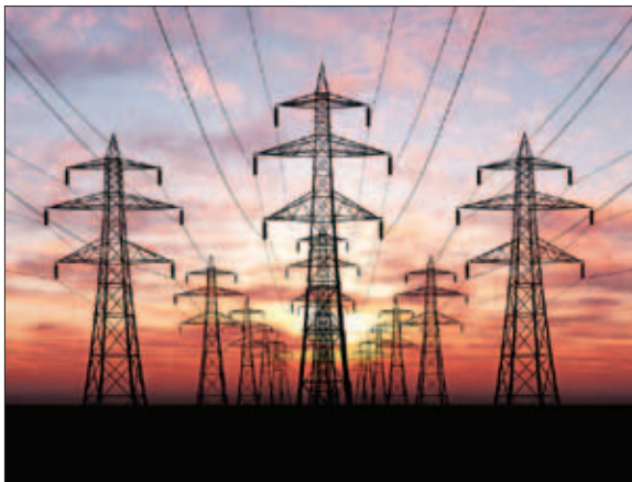
As U.S. energy producers adopt smart grid technology, it has the potential to bring benefits to domestic industry, particularly manufacturers and exporters of smart grid products and services. (photo © TebNad/iStock)
