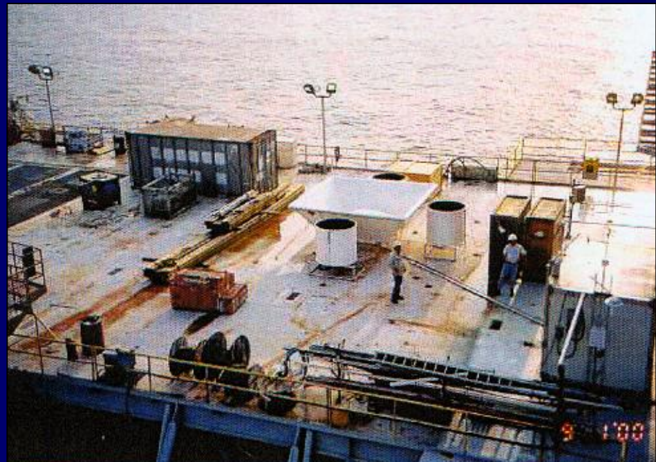
Radar Profiler/Radio Acoustic Sound System Installation on West Delta Platform
