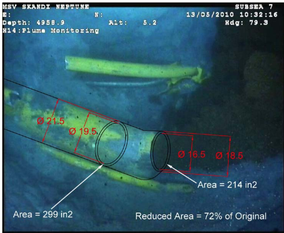
Figure 2: Riser Outlet Showing Its Reduced Cross-Sectional Area
