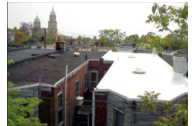
Philadelphia, PA reduced temperatures in row houses by installing cool roofs, which improves comfort for occupants and may help reduce deaths from heat waves. Baltimore, MD took similar steps following the success in Philadelphia.
