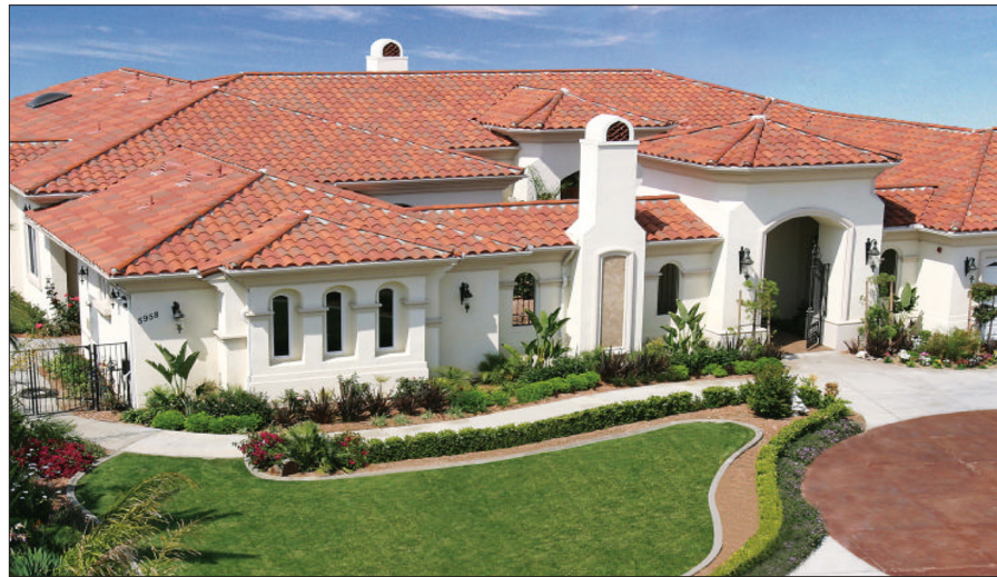
Cool roofing for residential buildings need not be white; cool colors are available for a number of roofing materials.
