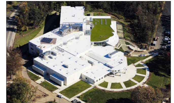
A white roof saves energy by strongly reflecting sunlight (high solar reflectance) and efficiently emitting thermal radiation (high thermal emittance).
