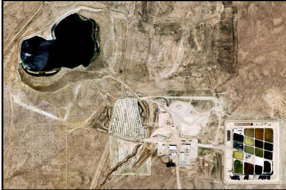
Figure 1: Sweetwater – Aerial View
