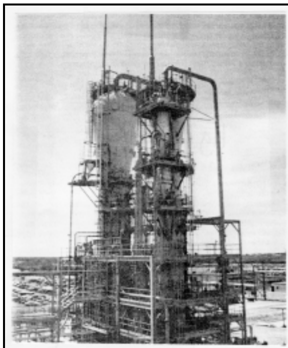
Figure 11: Fluid Reactors Used for Making Polypropylene
