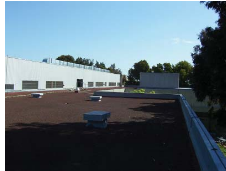
Example of a building that has no attic space. This is a roof with a mechanical penthouse.
