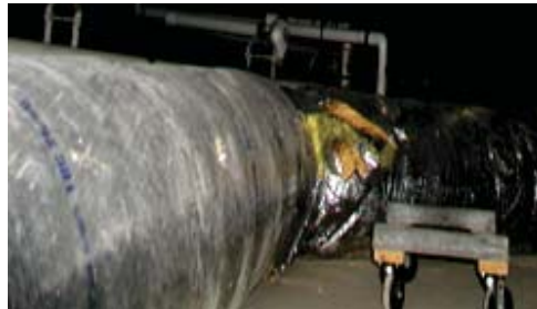
Crawl space inside opening of photograph at left. Note wheeled device used to lie on and roll within crawl space.
