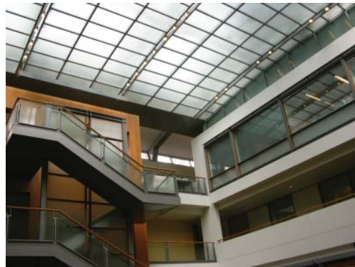
Example of a skylight above an enclosed courtyard.
