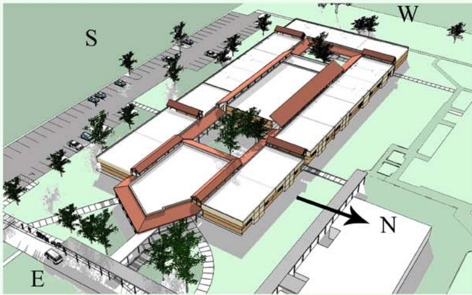
Materials: White roofs to reduce cooling loads
