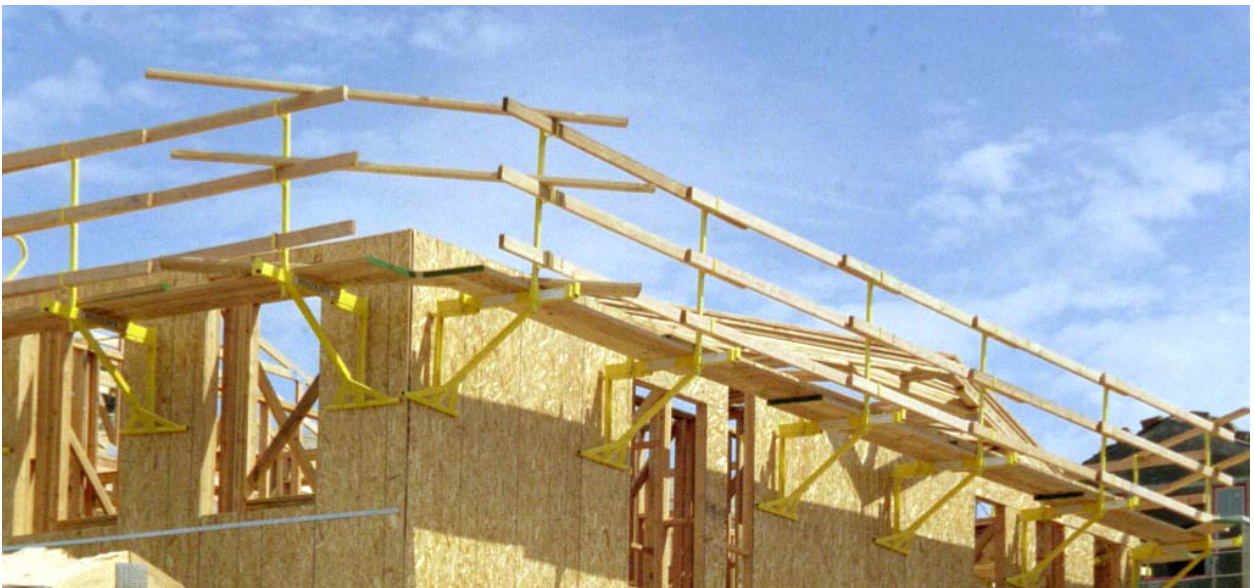
Figure 19 – A scaffold rigged for installing floor joists and floor trusses.
