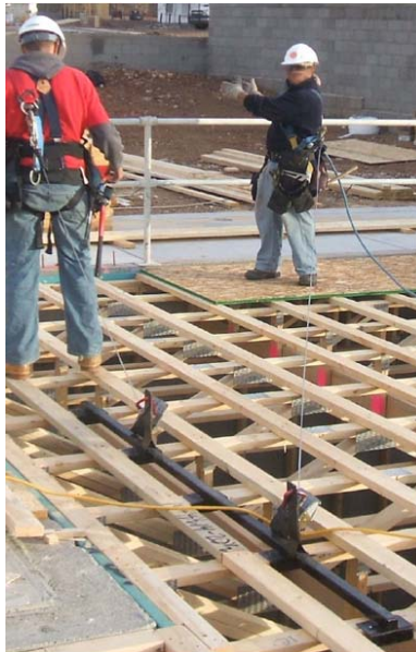
Figure 20 - Workers using a truss bracket anchor while installing a subfloor.
