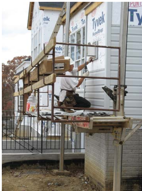
Figure 32 - A worker performing siding activities from a pump jack scaffold.
