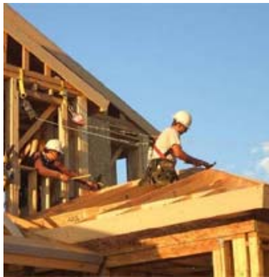
Figure 5 - Strap anchors providing anchorage for three personal fall arrest systems.
