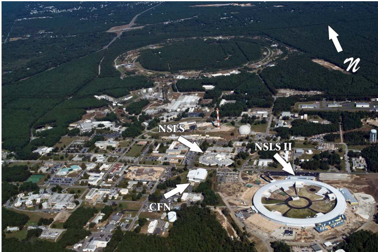
Figure 3.2: Aerial view of BNL (October 2011) showing the existing National Synchrotron Light Source (NSLS), the Center for Functional Nanomaterials (CFN), and the NSLS-II construction site.
