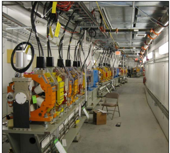
Figure 3. Completed cells 25 and 26 in storage ring pentant 1.
