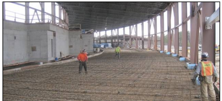
Figure 5: Preparations in pentant 5 for pouring the experimental floor.
