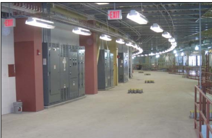
Figure 4: Signage installed, final paint touch-up on the pentant 1 mezzanine.
