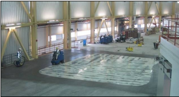
Figure 3: Pentant 1 floor being prepped for the application of floor sealer.
