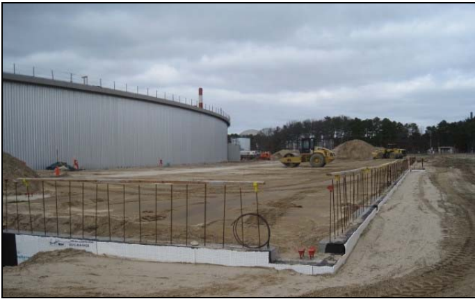
Figure 6: LOB 2 site being prepped for pouring the floor slab.
