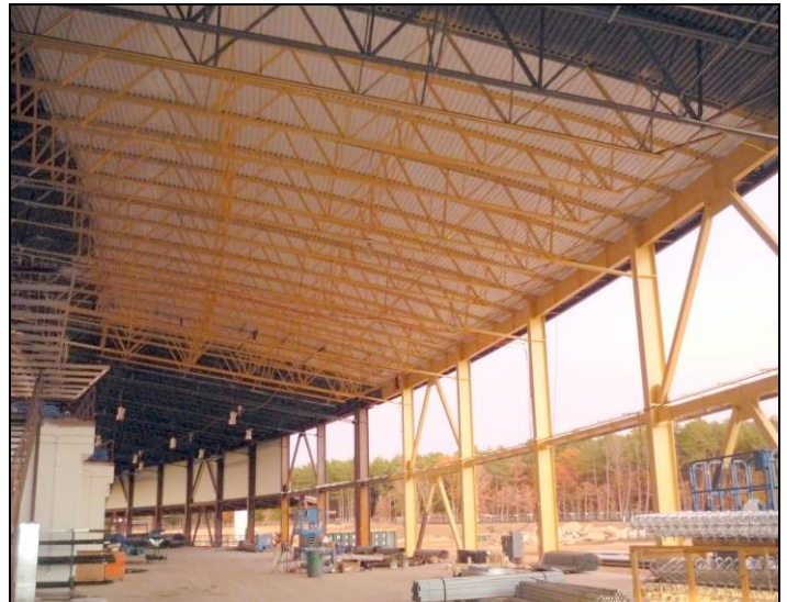
Fig. 7: Exposed steel and decking being painted in pentant 3.
