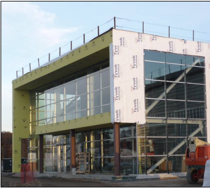
Fig. 8: The lobby becomes recognizable as the curtainwall glass is installed.
