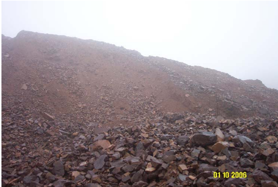
Figure 4.9 - Possible slope failure between Panel 100 and the full breach section
