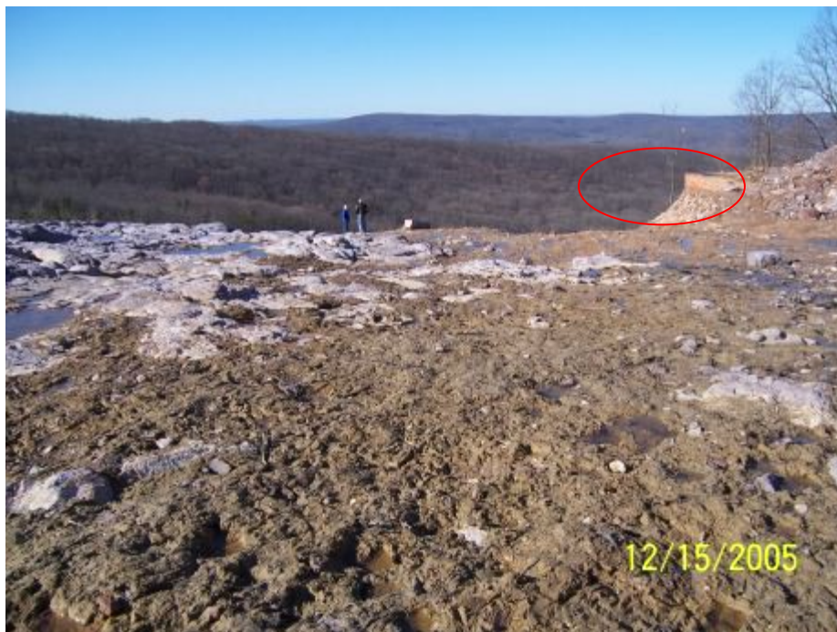
Figure 2.8 - Overview of area shown in previous photograph. Note washed out access road (circled).
