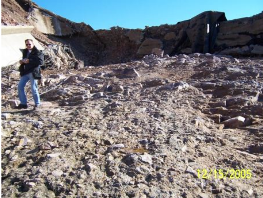
Figure 2.9 - Overview of area to the right of that shown in previous photograph. (See also Figure 2.4.) Note breach in background and toe of breach slope on left edge of photograph.
