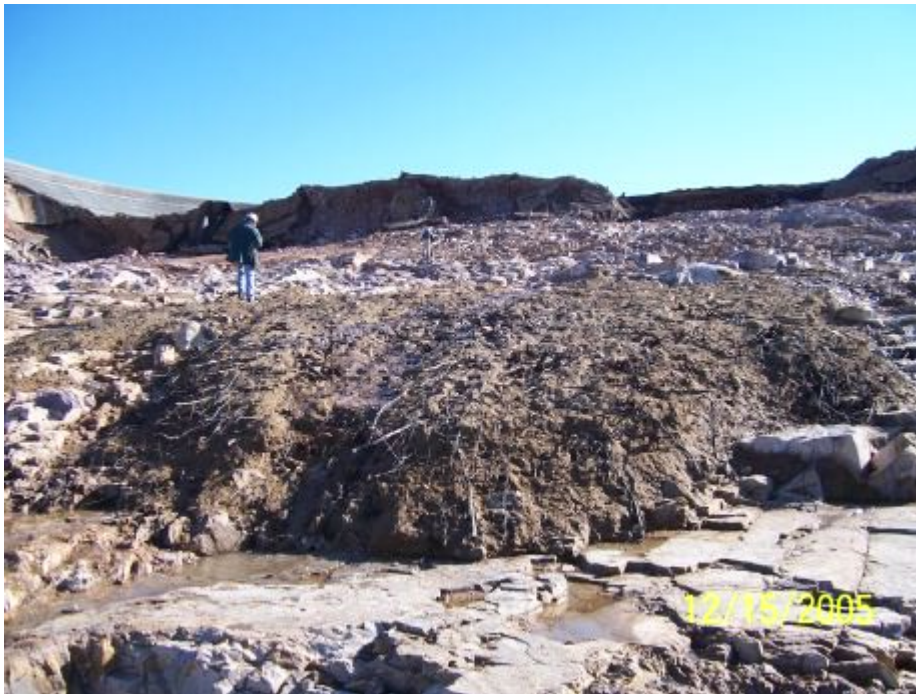
Figure 2.12 - Root-laden remnant native soil in breach area, resting on fresh rhyolite.
