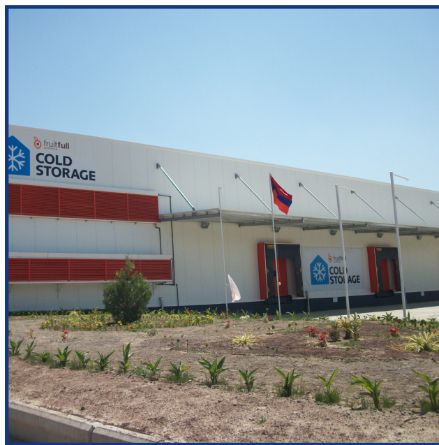
Zvartnots Airport Cold Storage Facility
