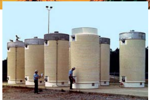
Water-filled storage pool and dry cask storage
