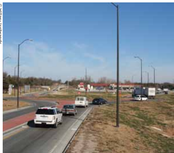
Traffic travels around a roundabout in Garnett, Kansas.
