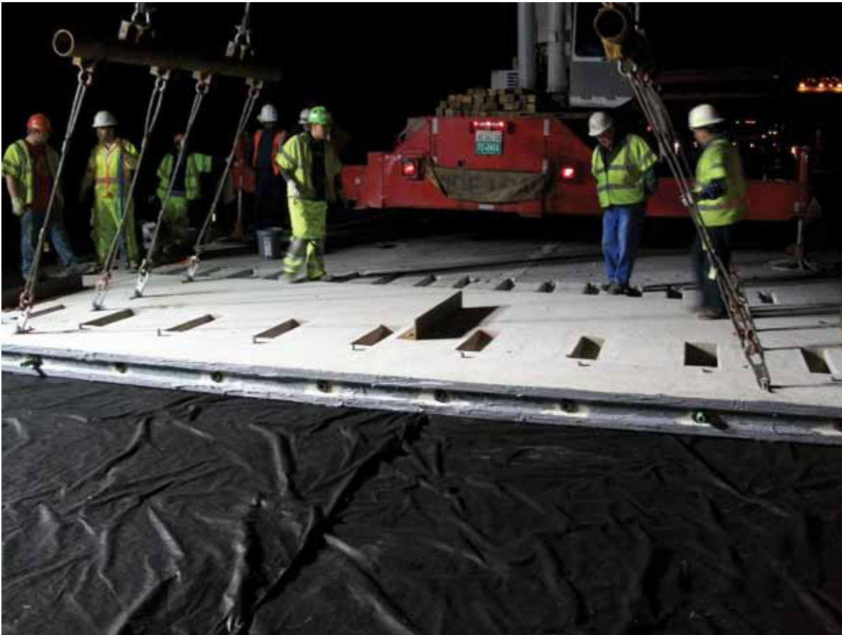
Precast, prestressed concrete panels are installed on I-66 in Fairfax County, Virginia, as part of a project supported by Highways for LIFE funding.
