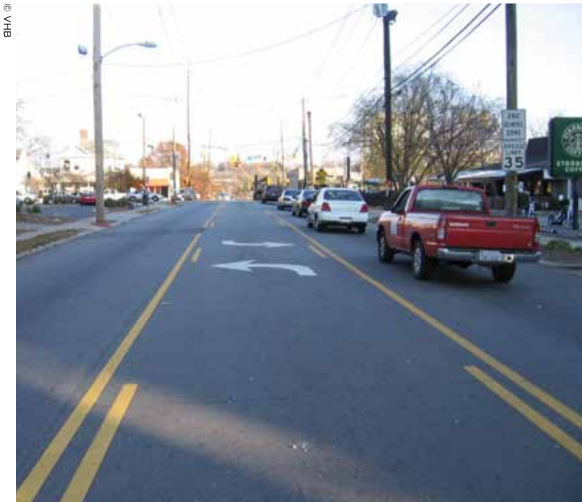
Safety improvement strategies can also include installing center two-way left-turn lanes on two-lane roads.
