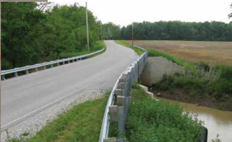
The Bowman Road Bridge in Defiance County, Ohio, was the first bridge in the world to use the Geosynthetic Reinforced Soil Integrated Bridge System (GRS-IBS).
