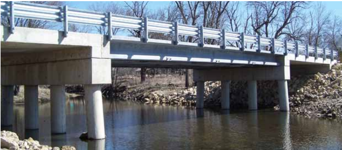
Ultra-high performance concrete pi-girders were used in the construction of the Jakway Park Bridge in Buchanan County, Iowa.
