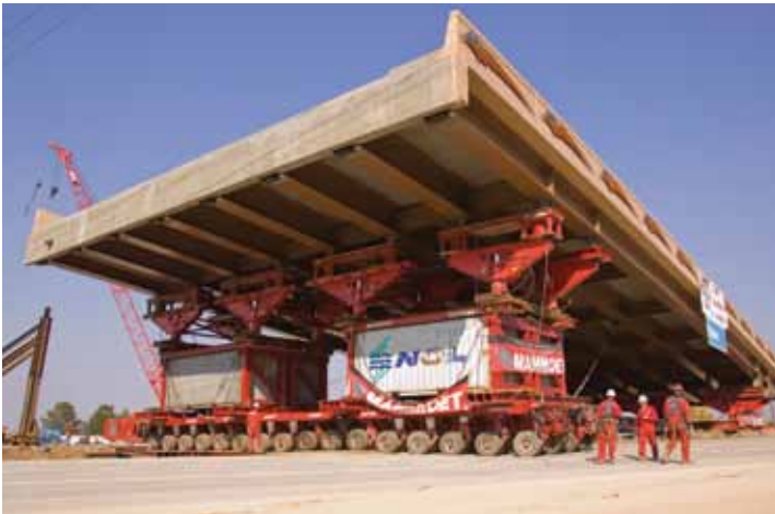
Utah is among the States now using prefabricated bridge elements and systems. Here, the prefabricated superstructure of the 4500 South bridge in Salt Lake City is installed.
