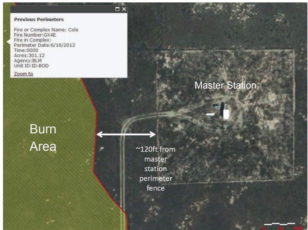
Aerial view of the Boise Master Station following the Cole Complex fire in mid-June.
