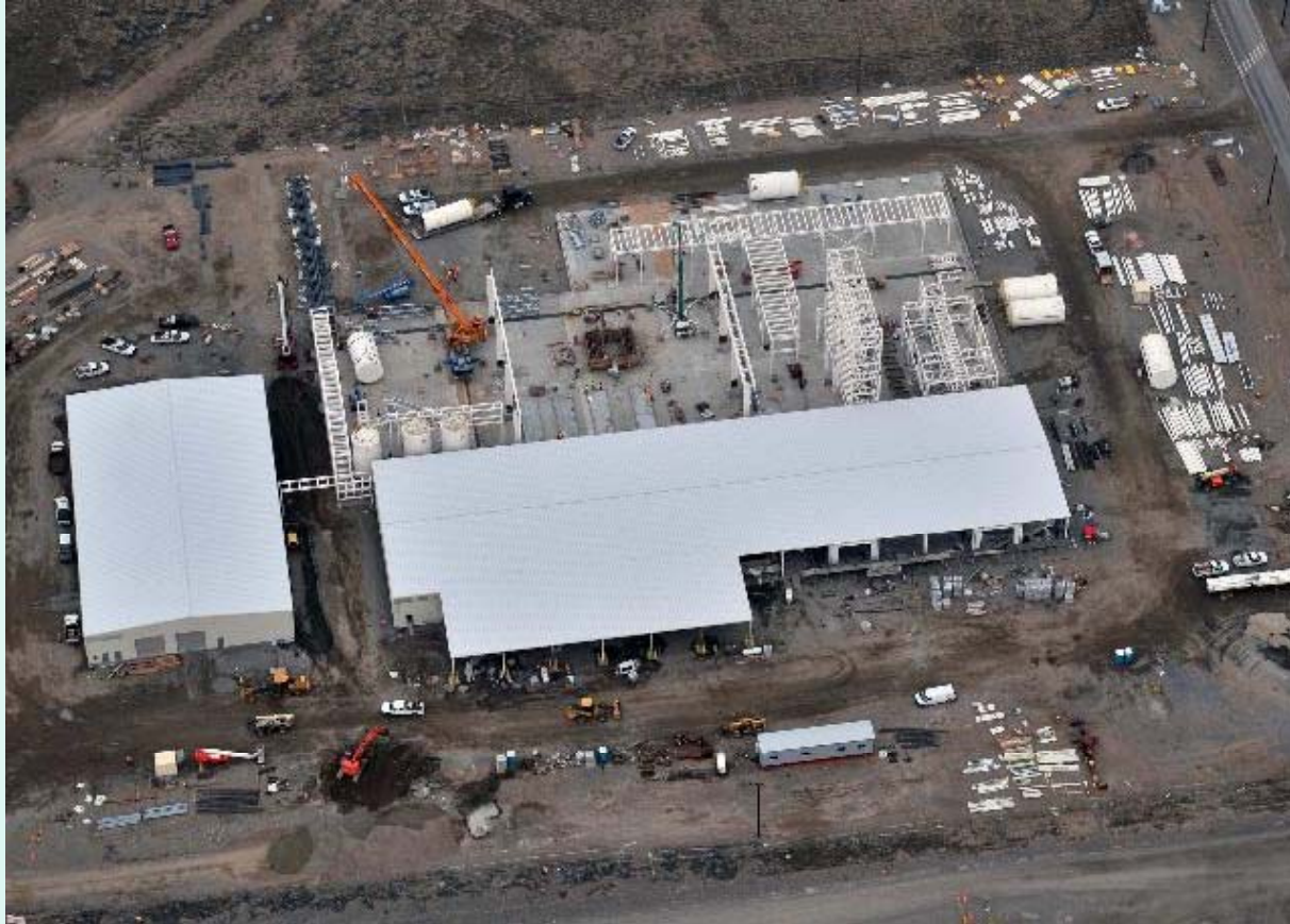
200 West Treatment Facility
